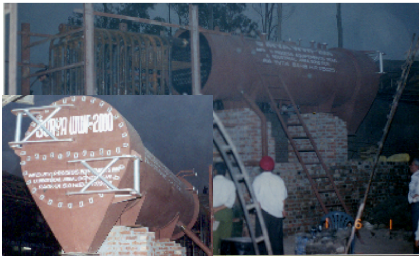
Waste Wood Fired, 2 Ton/Hr Boiler, under erection
